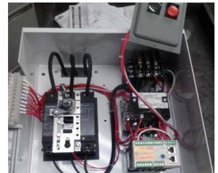
Unit after modernization
